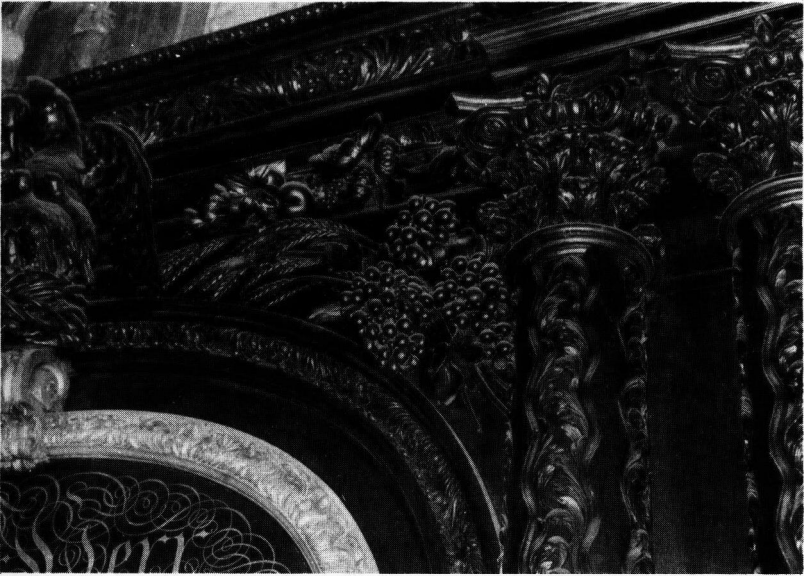
A detail of the reredos showing paired Corinthian columns and a spandrel filled with carving of wheat and grapes symbolizing the Eucharist—the communal taking of bread and wine. (Cluttons)
